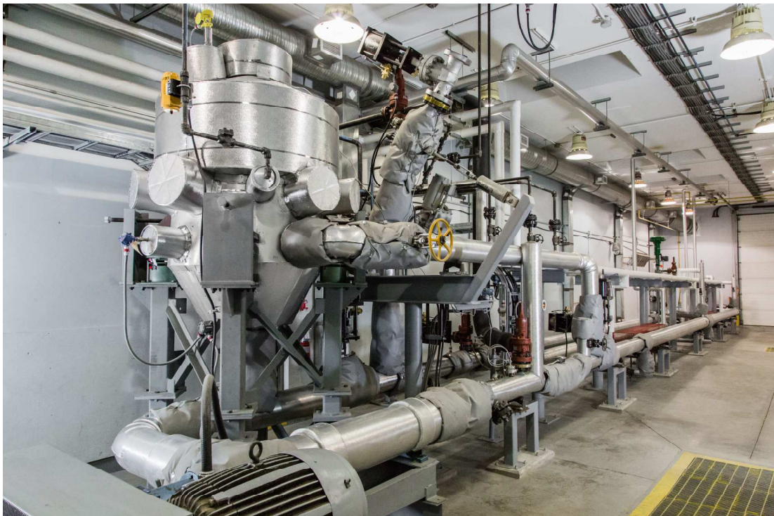
Figure 3.2 Closed loop pumping system (SASKATCHEWAN RESEARCH COUNCIL, 2014)
